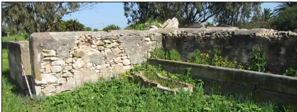
Figure 20: Feeding trough inside part of the historic farm complex at waypoint 237. Note the calcrete block walls.
