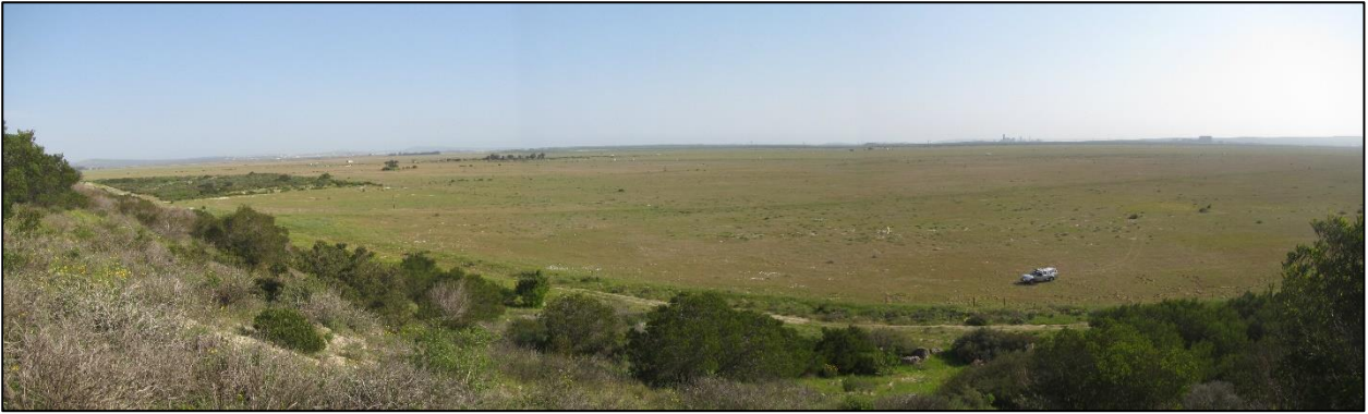
Figure 5: View towards the southwest across the proposed Alternative F site for the transmission substation. Alternative D lies in the background, while Alternative A is in the distance at far left of this picture. This view is from the berm along the western margin of the West Coast Fossil Park.
