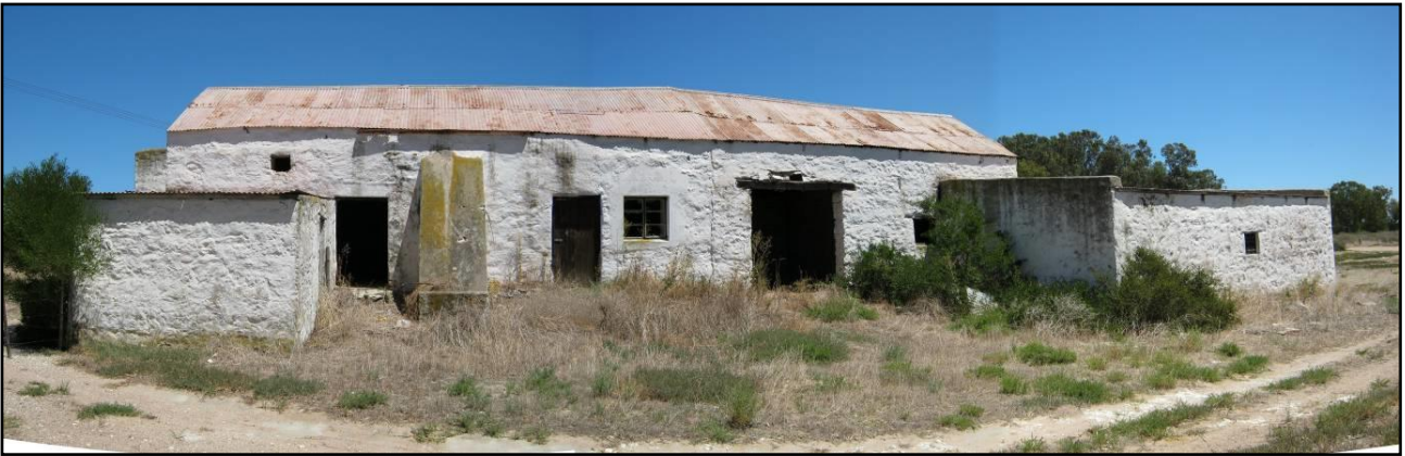
Figure 14: A typical stone-walled, tin-roofed vernacular farm structure on the farm Uyekraal 189 (Source: Orton 2011:figure 14).
